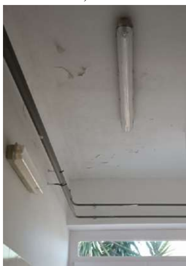
Bagno alunne piano terra pad. B
